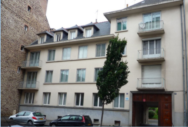
The house and the entrance porch, St-Hélier Street side
